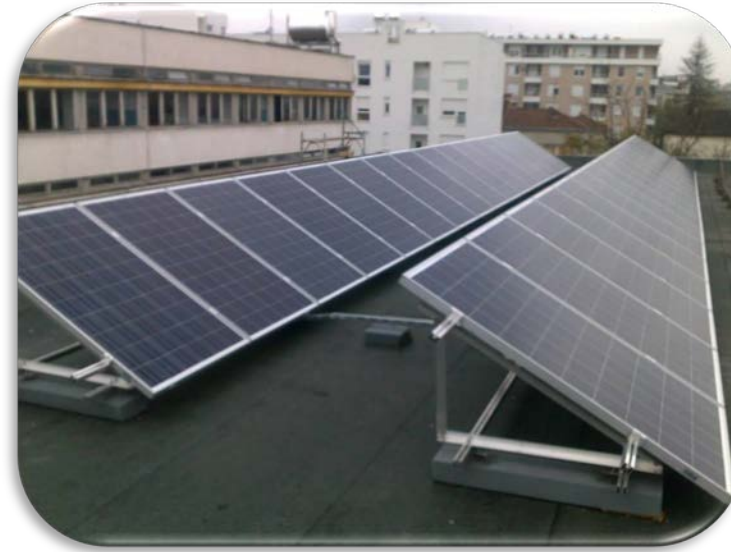
PV / solar panels installation
